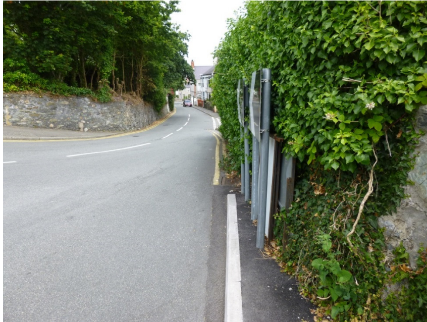
Photograph 18 – Gap in Footway Provision at Plas Road
