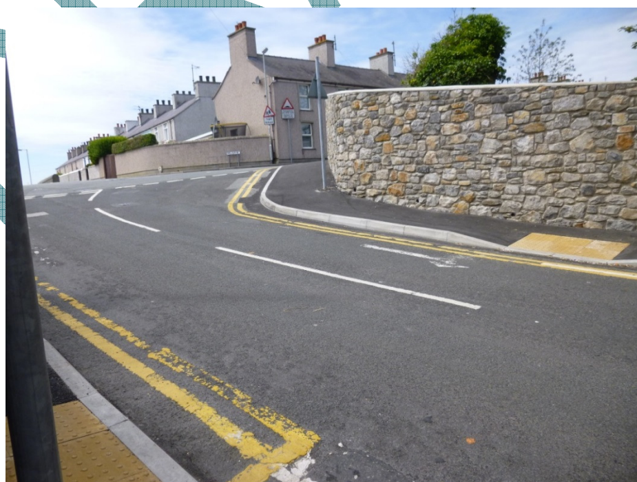
Photograph 9 – New Footway link from Gwynfa Hill to Mill Bank
