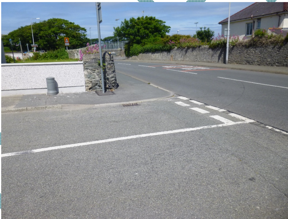
Photograph 17 - Drainage Gully in Line with Crossing at Maes Cybi (north)
